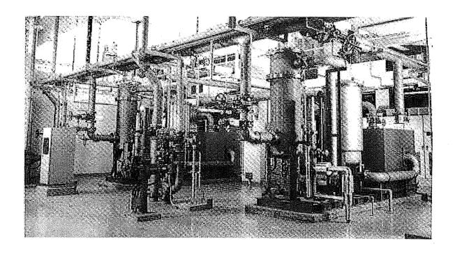
Contact time is usually about 10 to 15 minutes and ozone dosages of about 6.0 to 8.0 mg/l are usually sufficient to achieve effluent target bacterial levels.
